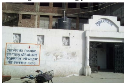
(Taimoor Nagar CTC after renovation)
